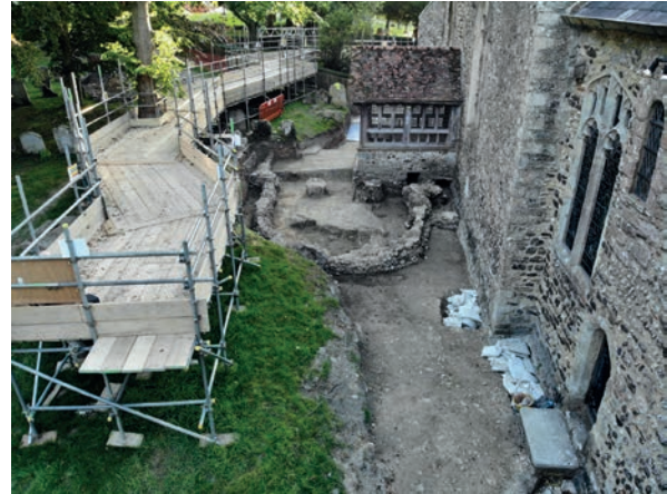
Fig 12. View of church foundations viewed from the east; the north wall of the nave can be seen running under the south porch. Photograph: authors.
