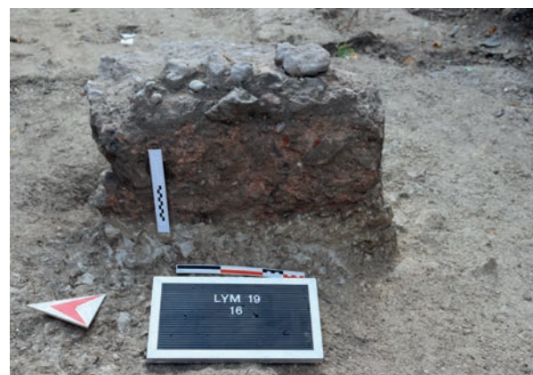
Fig 13. East face of south foundation pier (16) supporting cross-wall between nave and apse. Photograph: authors.
