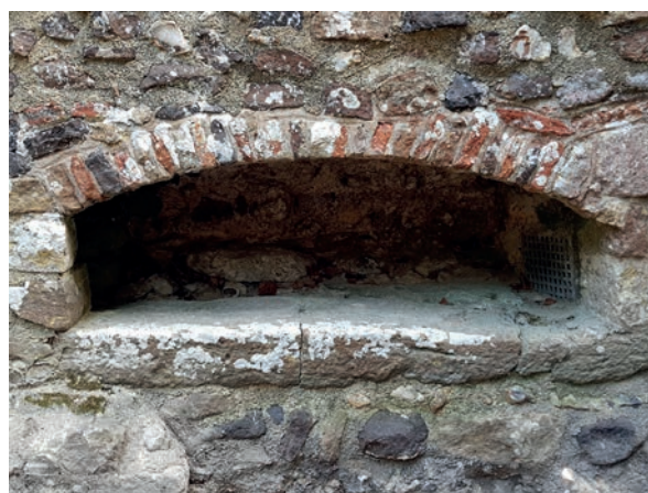
Fig 45. Detail of arched recess in south wall of nave. Photograph: authors.
