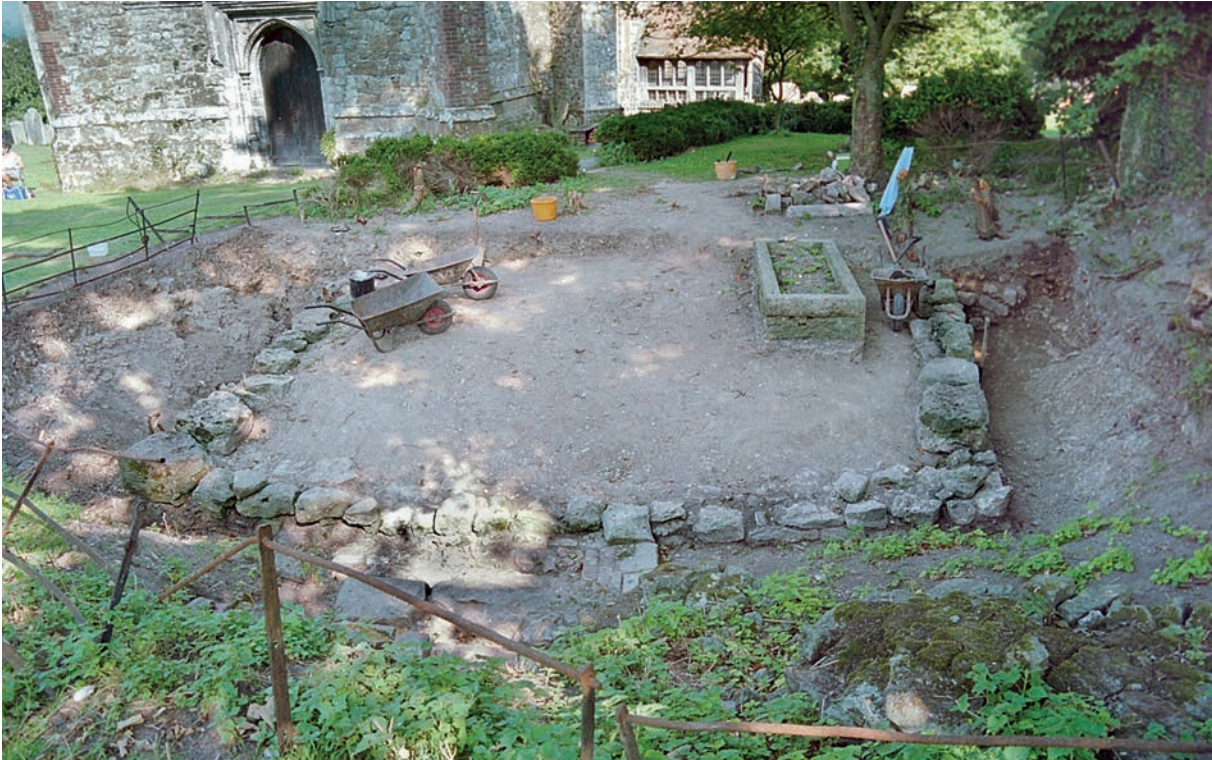
Fig 39. View of 1991–3 interventions in progress. Photograph: authors.
