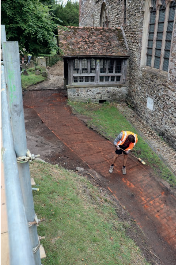
Fig 10. Former brick path to south porch revealed under its tarmac successor. Photograph: authors.
